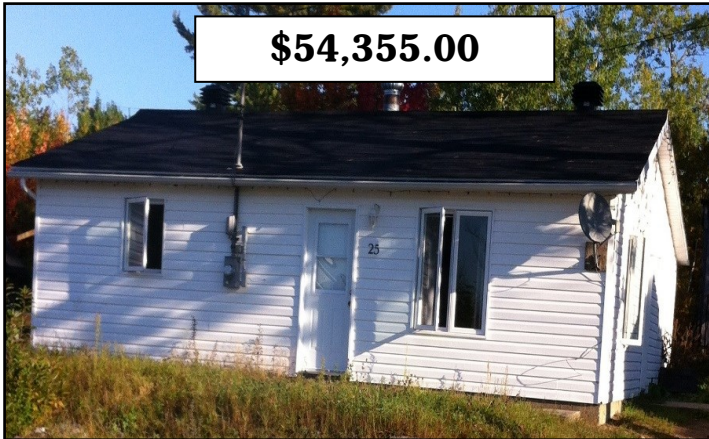
Located at 25 Amik Crescent
